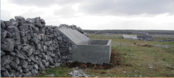
RAINWATER CATCHER USED TO BRING WATER TO REMOTE PARTS OF ARAN FARMS. Source: Amanda Browne
