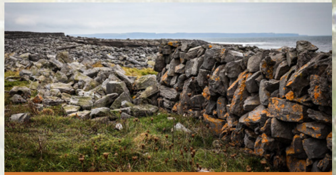
STONE WALL REPAIR. Source: Conor Coyne
